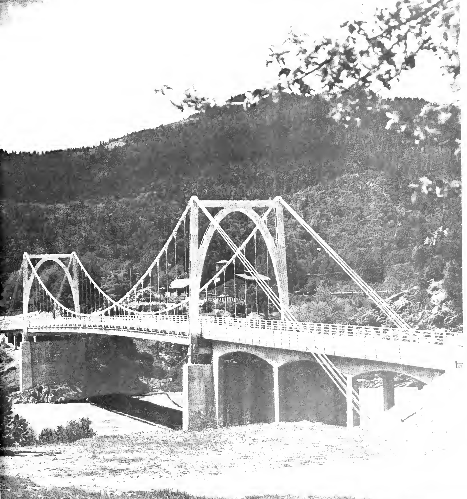
NEW BRIDGE ACROSS KEMASH RIVER AT ORLEANS, HUMBOLDT COUNTY ON STATE HIGH ROUTE 29 THAT WON FIRST PRIZE IN NATIONAL DESIGN COMPETITION (SEE ARTICLE IN THIS ISSUE)
